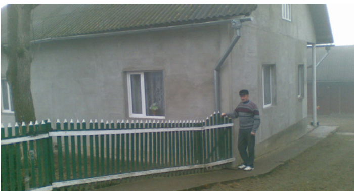
The house of the Ukrainian family from Velesniv before the reconstruction and after outer insulation and windows replacement.
